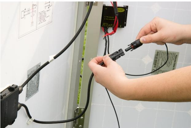
**Step 4:** Connect Panel A's positive (top) plug to the charge controller's positive (red) plug.
