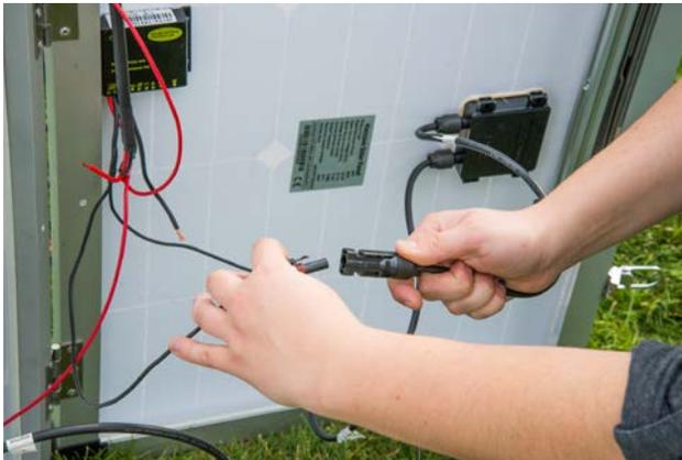
**Step 6:** Connect Panel B's positive (bottom) plug to the charge controller's positive (red) plug.
