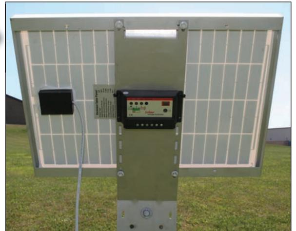
Once panel is secured, attach a solar charge controller (MSC5LVD) to the bracket with zip ties (included) using the four small holes.
