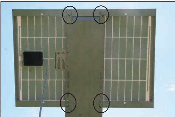
Center the panel and then secure it to the bracket with four self-tapping screws (included) as circled. Use the slots on the bracket to determine screw placement.
